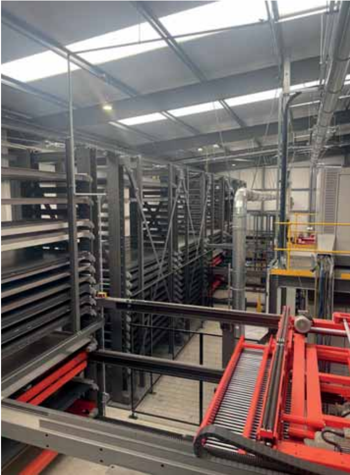
Material storage within the loading system
