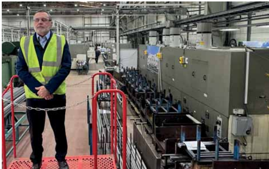
Darren from Crittall Windows with Filtermist extraction systems on specialist machines to the right as well as on CNC machines in background.
