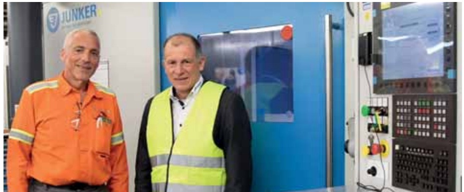
From left to right: Thomas Bender (foreman, production-related workshops at Saarstahl, Burbach) and Waldemar Neumayer (regional sales manager, JUNKER) in front of the Lean Selection Shaft at the Burbach plant, Germany.
